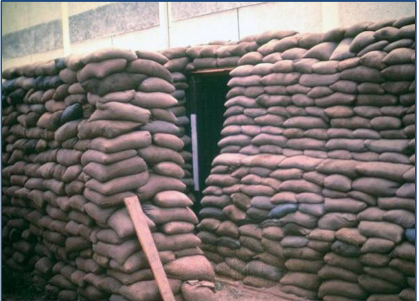
The bunker just outside the back door to the main building.
