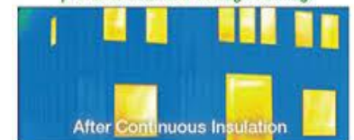
Adding exterior continuous insulation prevents heat flow through framing.
