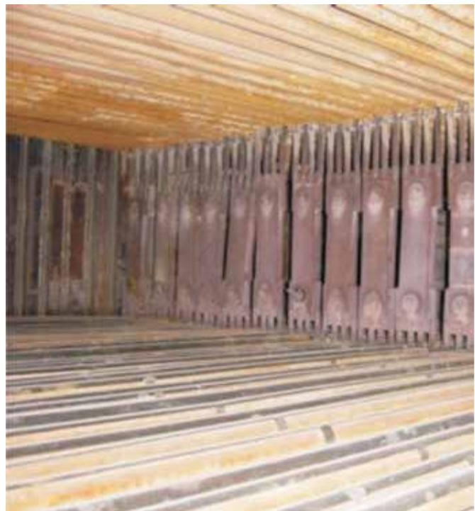
Fig-2: Support plates separating two assemblies of coiled tubes.
