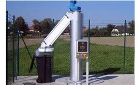
The RoK 4 screen vertically lifts the screenings, and dewater and compacts them at the same time. The compacted screenings are discharged into a container or endless bagger for further disposal thus eliminating odour nuisance and pump failure due to clogging.
