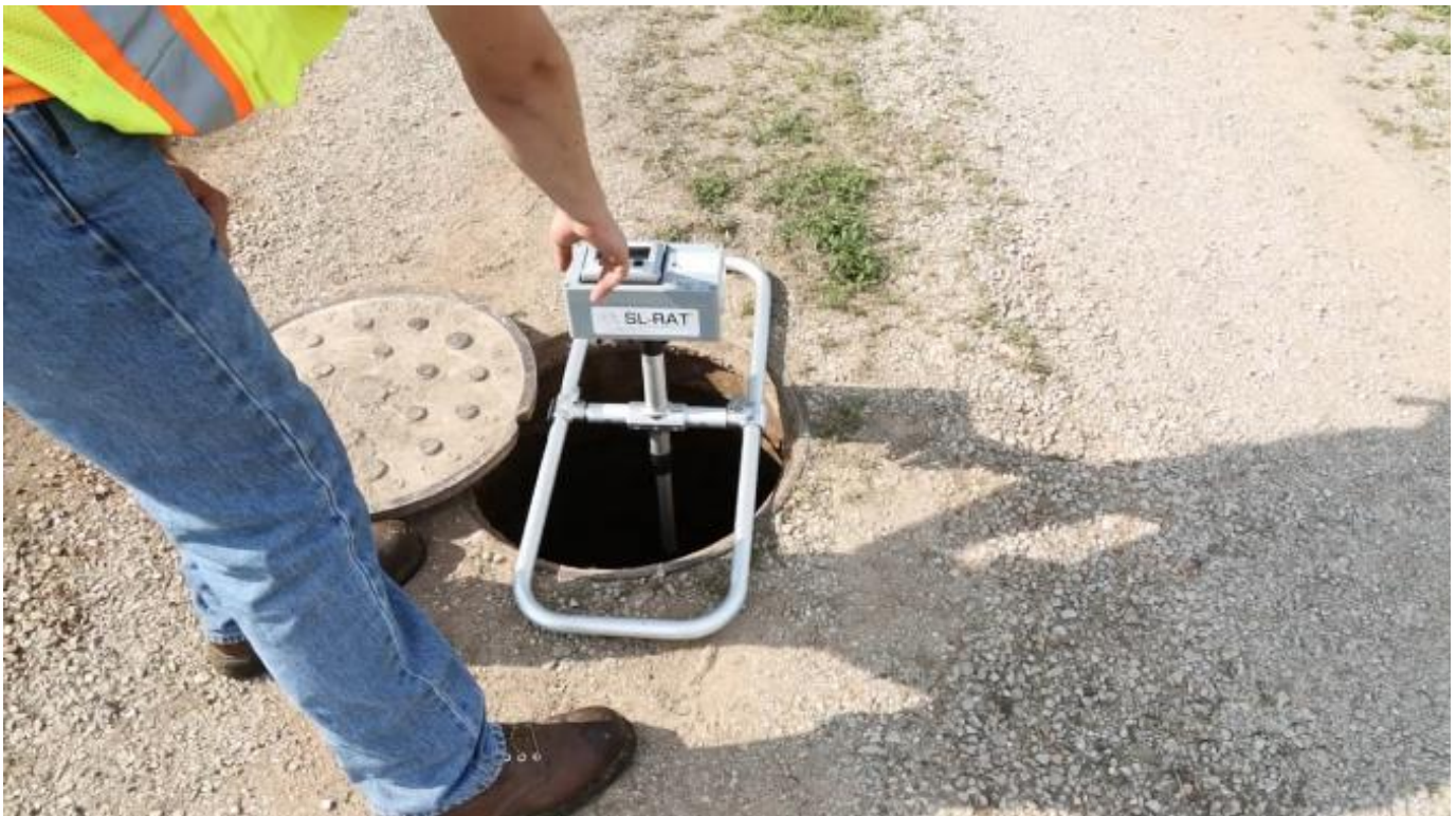
Figure 2-5: SL-RAT Performing an Acoustic Sounding Test
