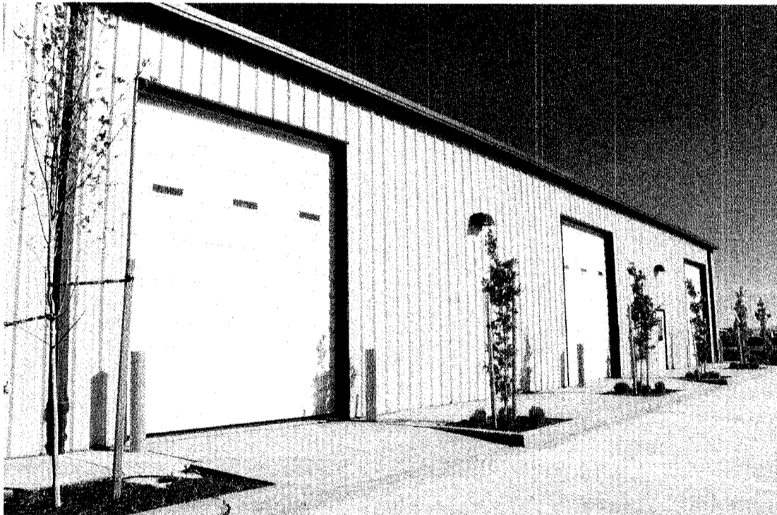
Alpine Power Systems has leased the Flex building. Welcome Alpine!
