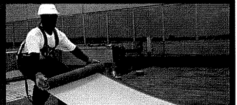
Roofing & Sheet Metal
