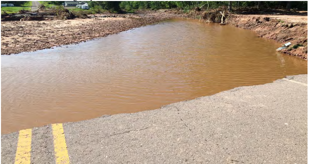
Photo 5: View to South. Post 2016 disaster event. Disaster rechannelized Oronto Creek and breached Highway A.
