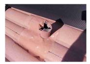
•The valley flashings need to be cleaned and kept clean. E.G. There is debris in the valley on the west side roof that needs to be cleared.
