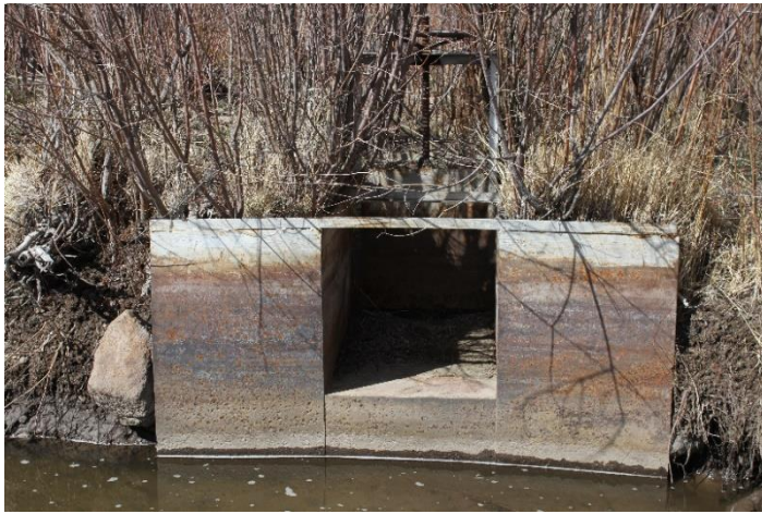
Headgate looking downstream
