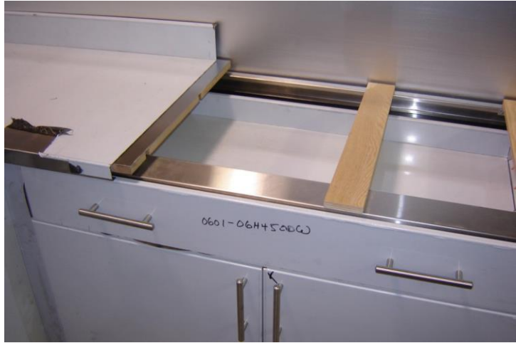
Left side has tongue extending beyond edge of countertop. Right side has stainless steel overhang
