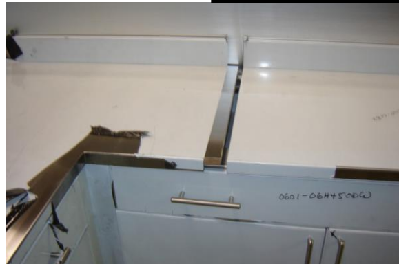
Use drawbolts and leveling plates to install top.
