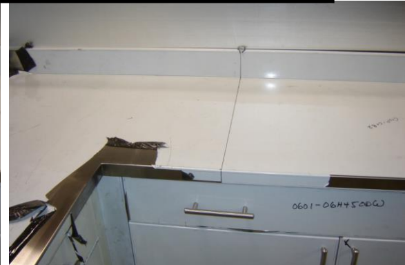
Use drawbolts and leveling plates to install top.
