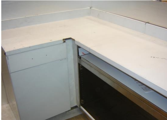
Remove doors and drawers for access to underside of countertop.
