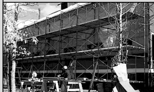
Restoring the Recreation Hall.
