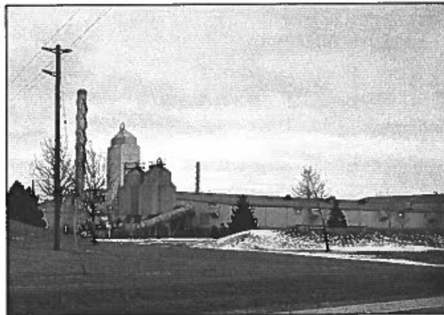
The Brampton Brick facility, on Highway 10 at Wanless Drive.
