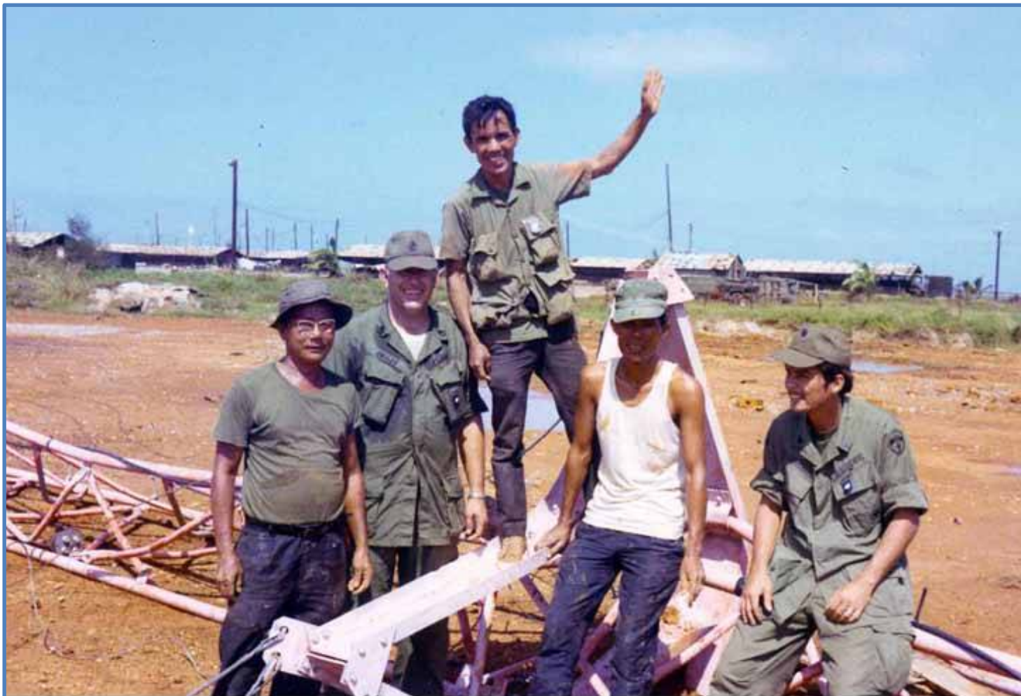
With some of the AFVN "local hire" tower crew taking down the Chu Lai tower.
