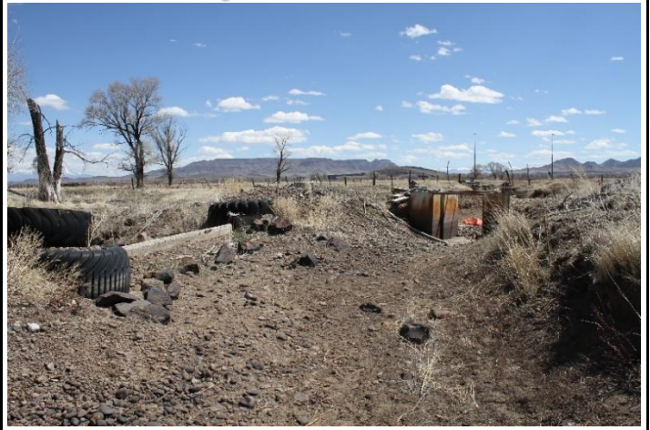
Headgate and diversion dam
