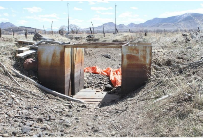
Headgate looking downstream
