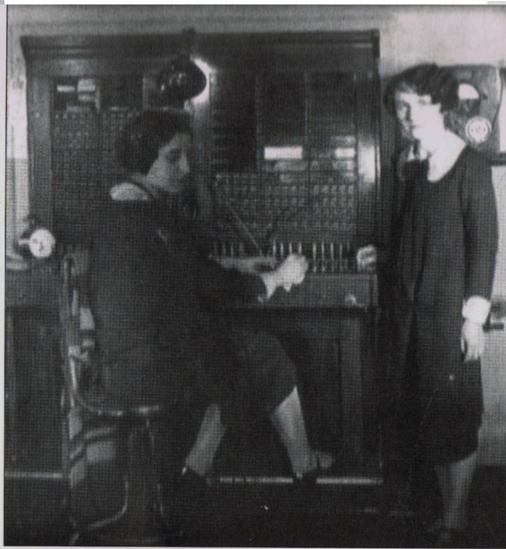
Progress continued to come to Brooklyn Township as pay stations were finally closed in Osseo in 1915. Booths were removed and connections were made to the switchboard of the local Rural Telephone Company, now connected to the Northwestern Telephone Company. Mildred Smith (left) and Myrtle Engles were switchboard operators in 1926. (Courtesy of Osseo Preservation Society.)
