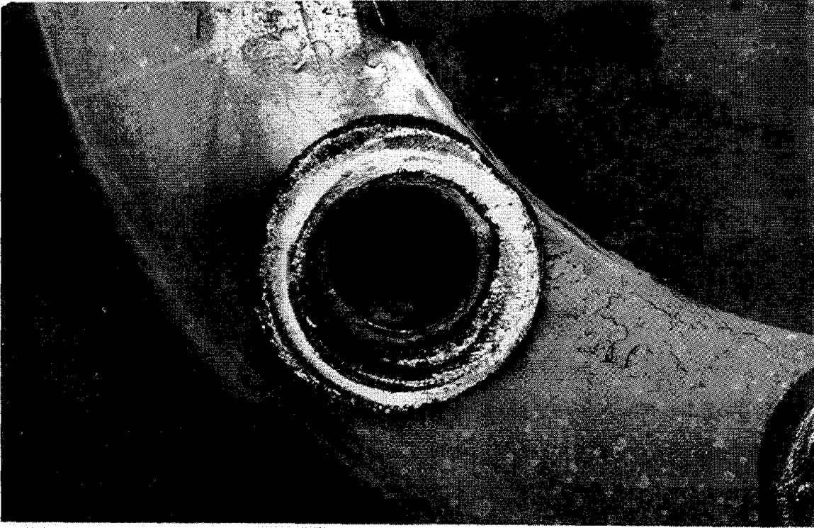
Figure 8.--Mounting face wear on outboard wheel assembly.
