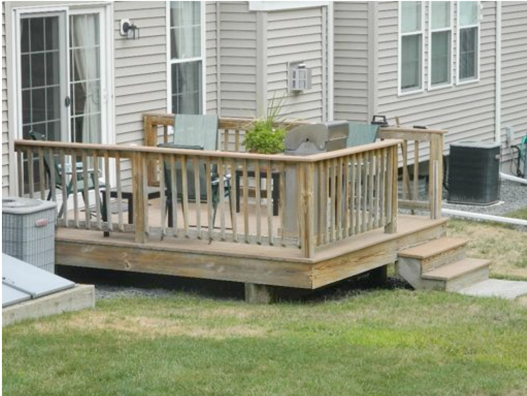
TYPICAL GRADE-LEVEL OPEN WOOD DECK
