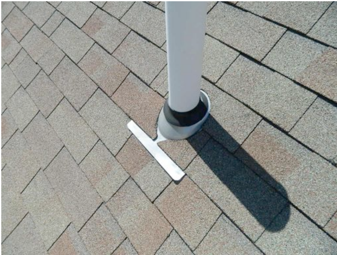
TYPICAL NEOPRENE/ALUMINUM PIPE FLASHING
