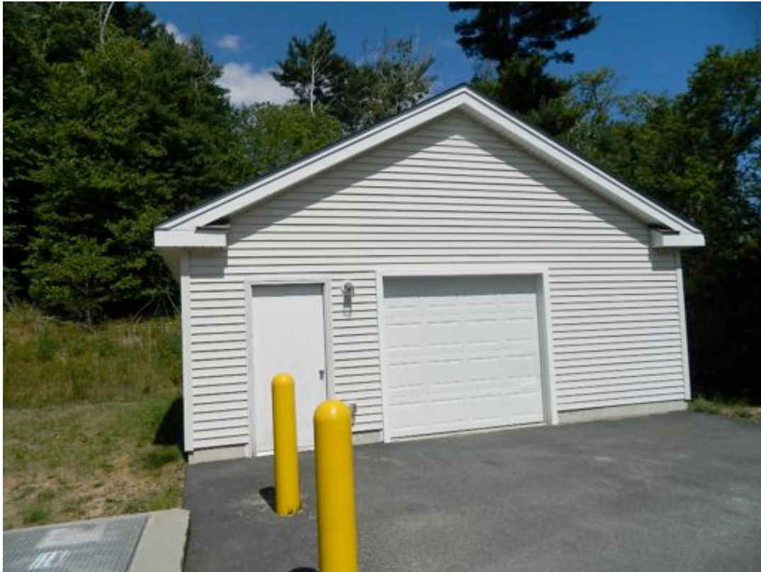
OVERVIEW OF THE WWTP AREA STORAGE GARAGE
