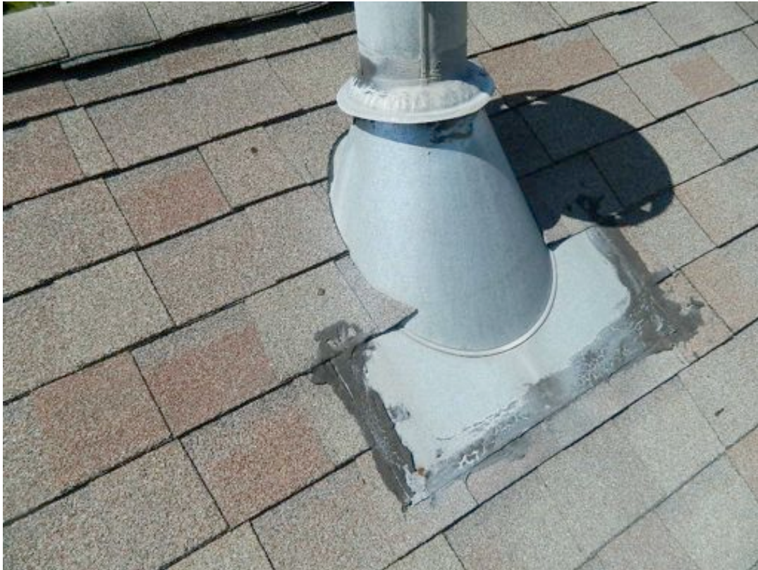
TYPICAL TYPE B GAS VENT STACK FLASHING
