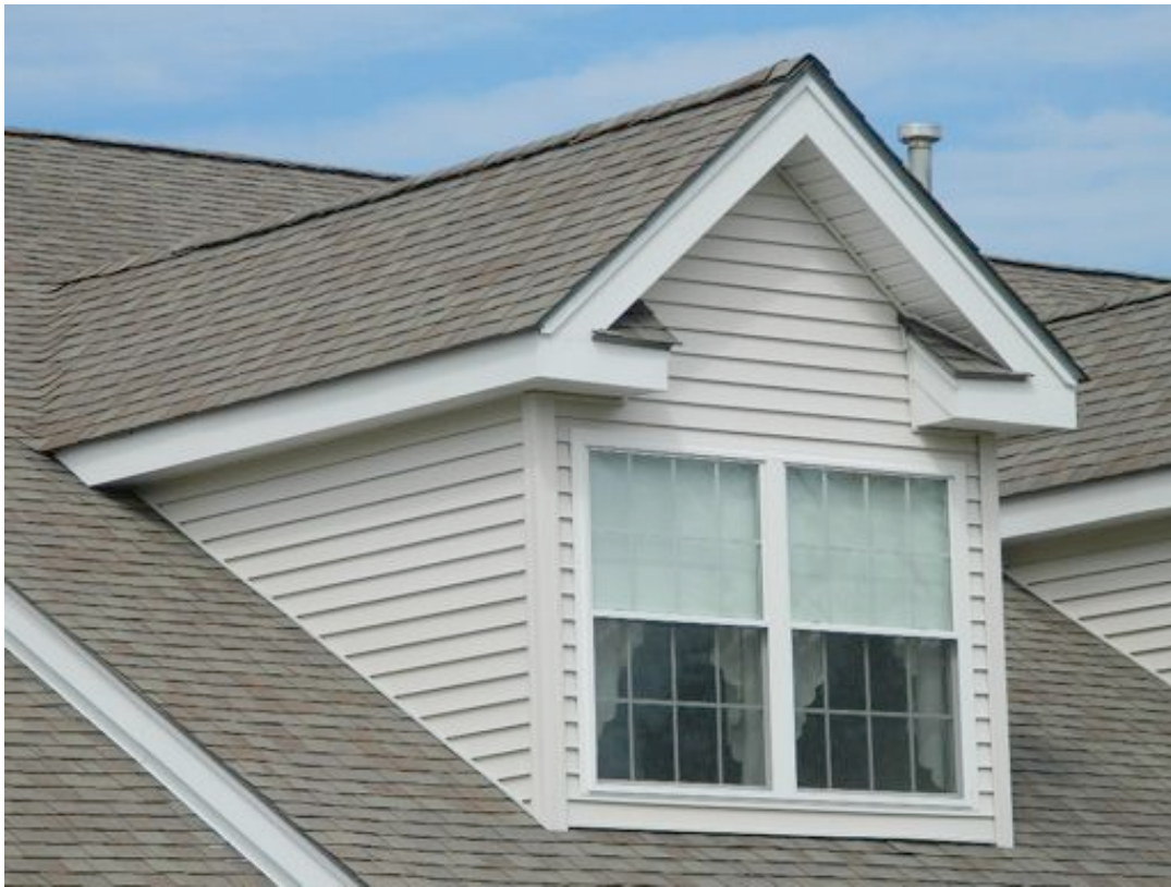
TYPICAL ABOVE-ROOF WINDOW DORMER
