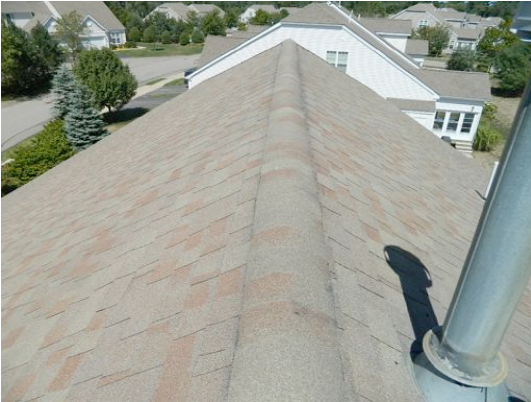
TYPICAL SHINGLED-OVER RIDGE VENT
