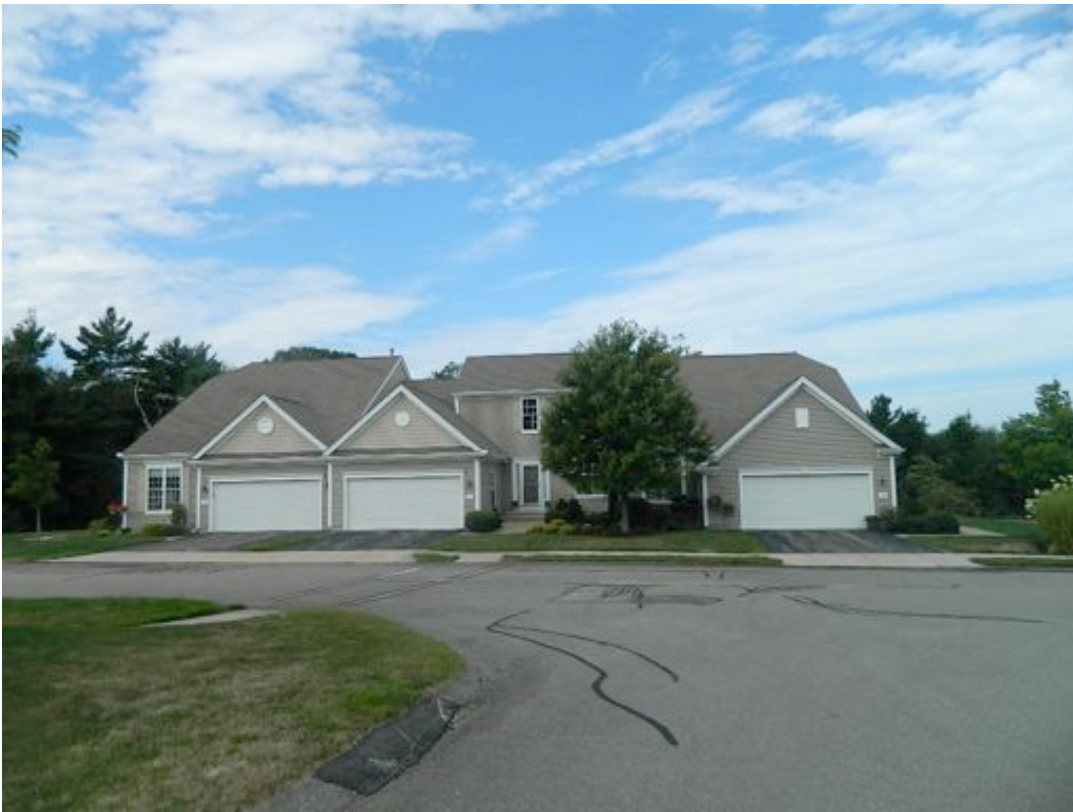
FRONT OVERVIEW OF A TYPICAL BUILDING AT SPYGLASS LANDING
