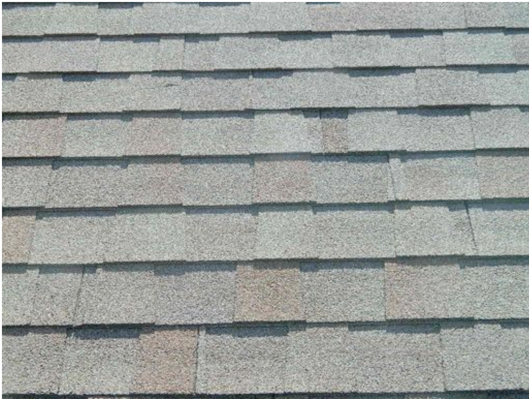
FIBERGLASS-REINFORCED RANDOM TAB SHINGLES
