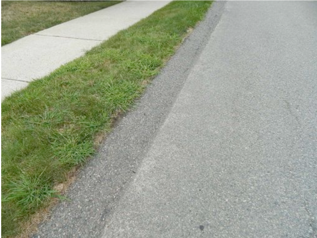
TYPICAL EXTRUDED CAPE COD BERM
