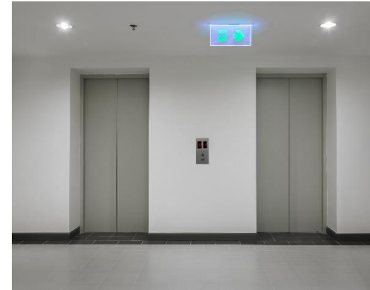
Elevators and Lobby Area
