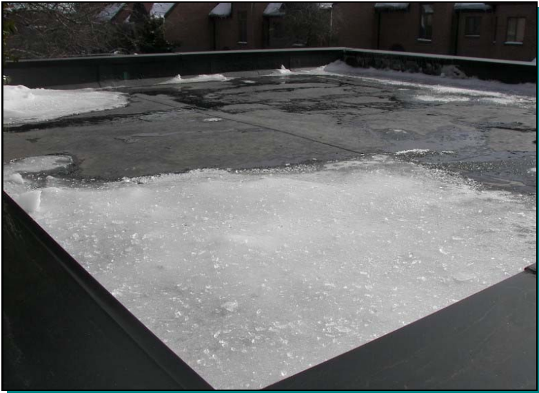
Typical EPDM roof at garage
