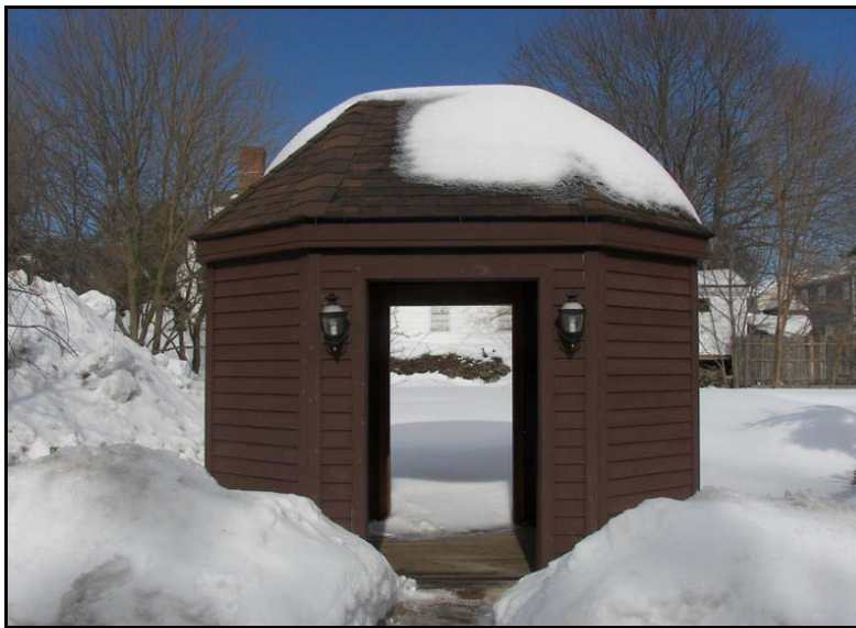
Mailbox station shelter
