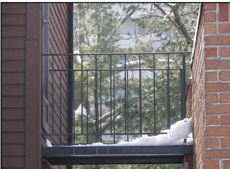
Metal bridge assembly
