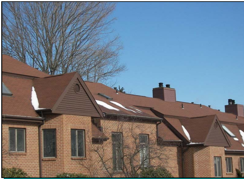
Asphalt shingle roof overview
