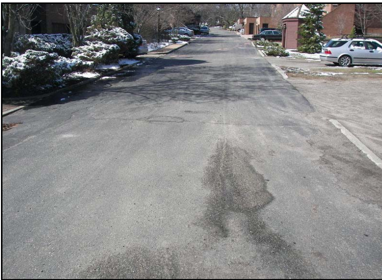
Asphalt pavement overview
