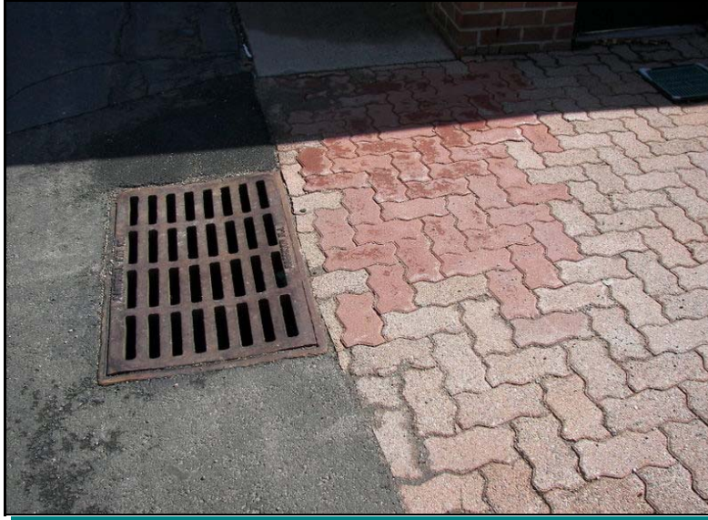
Example of previous partial brick paver replacement
