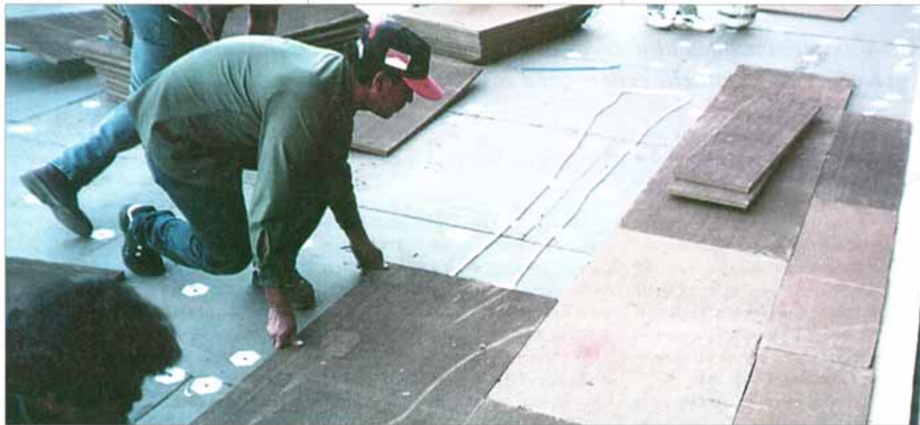
Crews attached rigid insulation boards using a foam adhesive.
