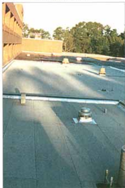
Prefinished galvanized steel flashings enhance the roof's aesthetic appeal.
