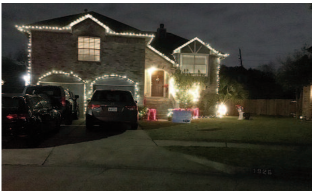
Section Three - 1926 Northcliff Place
