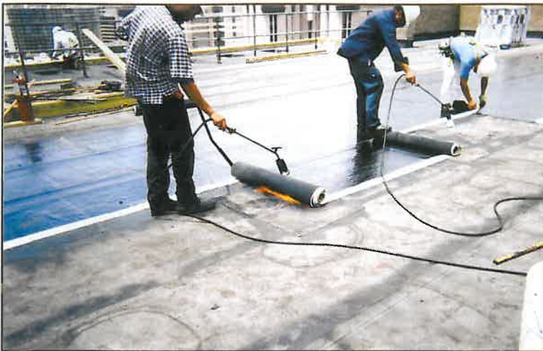
Installation of membrane.
