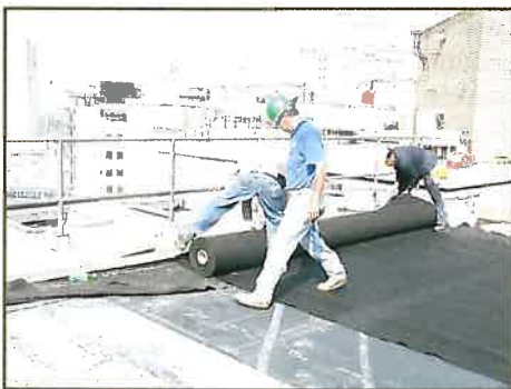
Installation of drain board.
