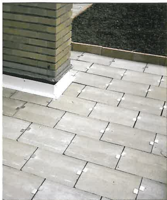
Typical wall flashing.
