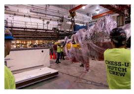
To reduce installation time at CHESS, all Front-End components were assembled onto a single support beam and precisely aligned. The fully assembled FE's were then tested, pumped down, and baked-out prior delivery to CHESS. Off-site alignment at ADC allowed for a final installation which only required positioning of the support beam, and not each individual component. Off-site pumping down and baking also aided in reducing beamline downtime.
