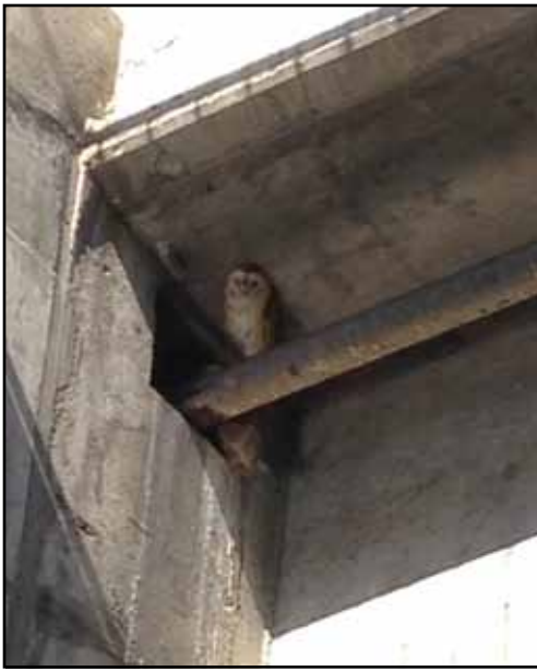
Owls under the Foster City Blvd. Bridge
