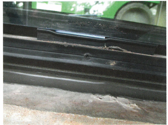
Figure 6. Plastic shim between setting block and glass lite.
