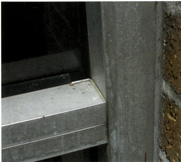
Figure 13. Photo of gap between ends of abutting gaskets at interface of vertical and horizontal mullions.
