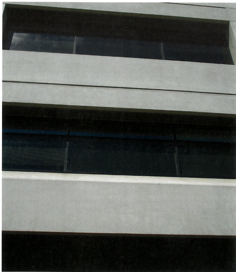
Figure 19. Photo of sealant joints in wall panels intersecting joint around window frame.
