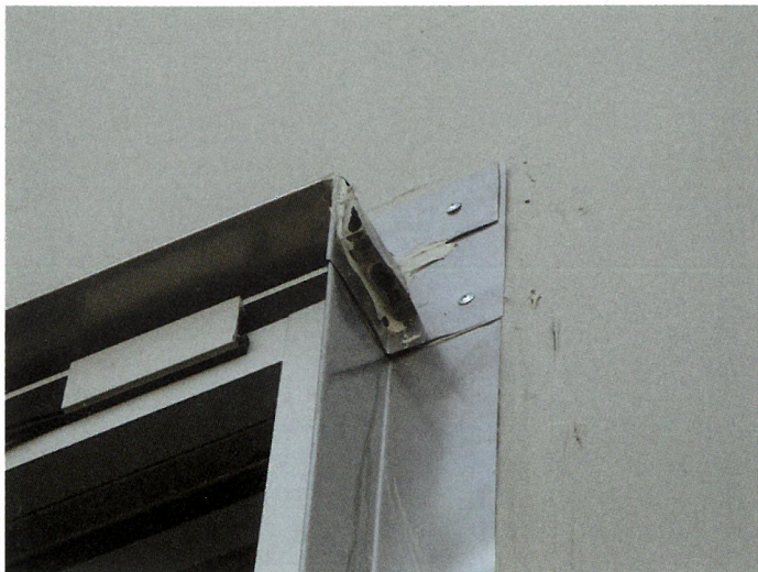
Figure 15. Photo of sheet metal weathering flange corner lap.
