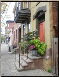
Row House in Troy, NY
