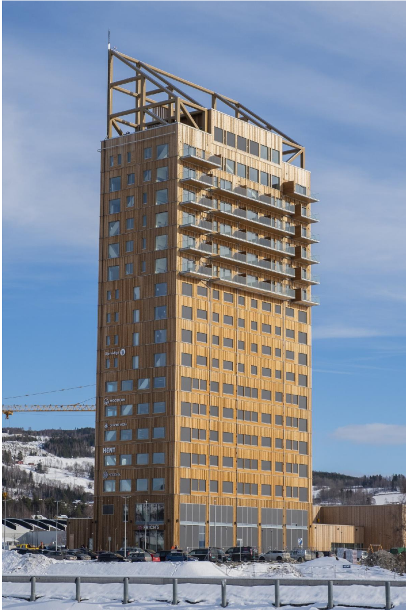
Above: 280' timber framed building in recently completed in Norway.
