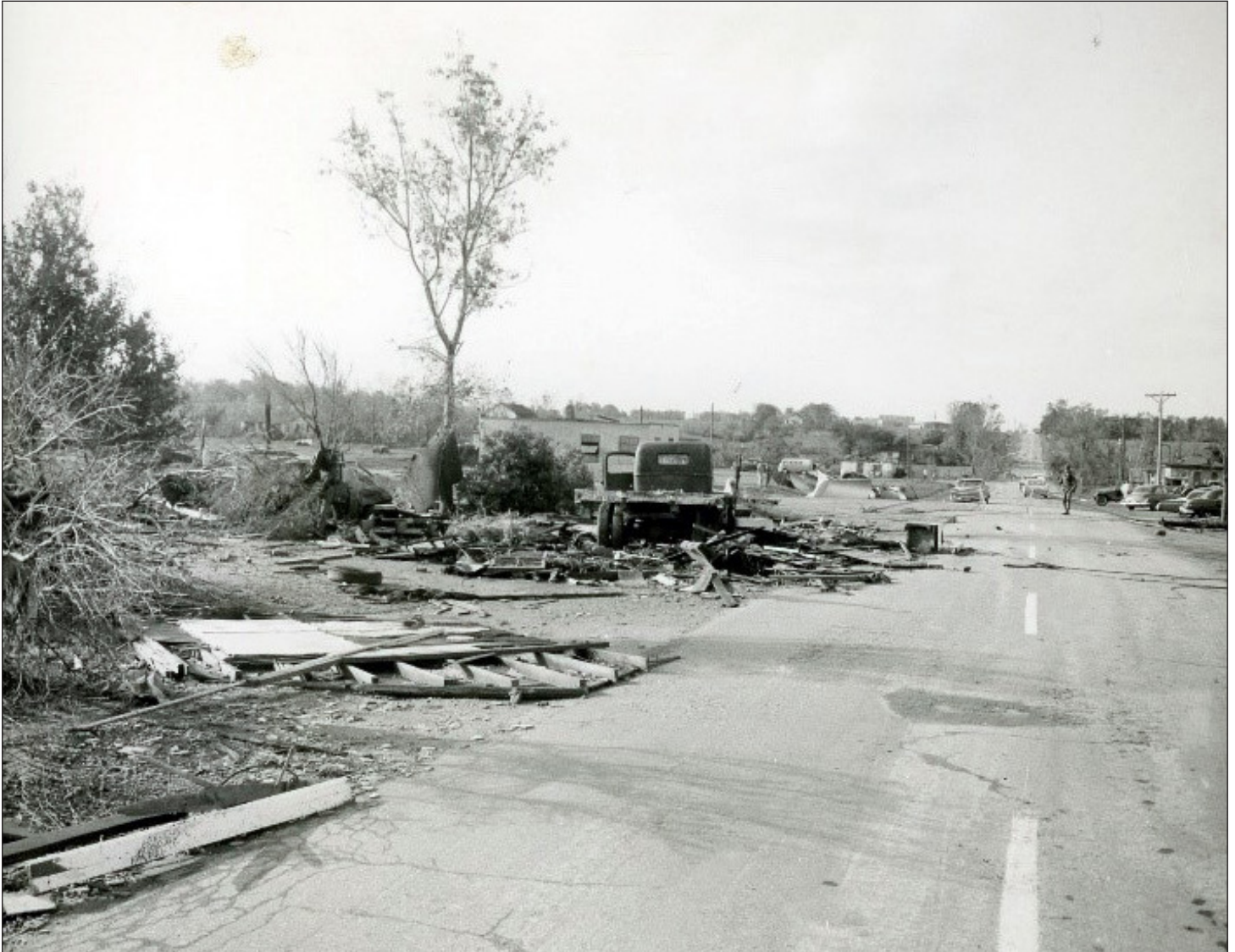
THIS PHOTO SHOWS THE TORNADO'S DESTRUCTION along Ohlman Street in Mitchell.
