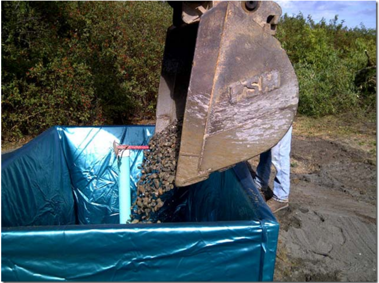
Filling Glendon basins with gravel media.
