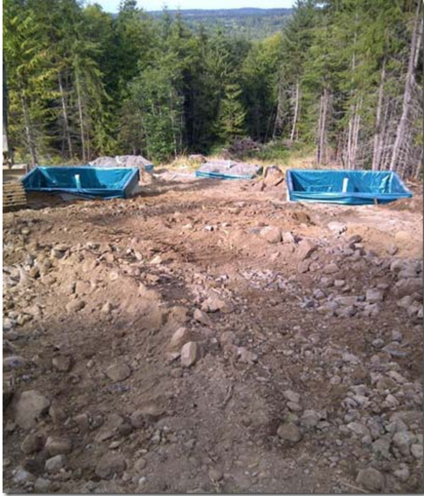
Building Glendons on a hillside.
