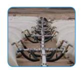
Using an SEI-engineered system, the tanks are filled with fuel through an innovative network of manifolds and pumps. Tanks can be isolated into groups of four or filled individually, if required.
