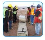
Using 6-8 personnel, unfolding an Arctic King<sup>TM</sup> tank can be accomplished quickly and easily. Very little training is required, especially once the team experiences the set-up of the first tank. With a team leader in charge, straps are removed and the Arctic King<sup>TM</sup> tank is soon deployed into its new location.
