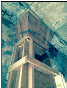
Figure 3: Powerhouse interior column forming
