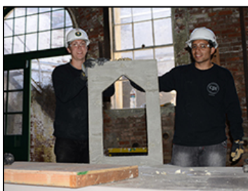
Figure 8: Custom precast panel for concrete railing repair project
