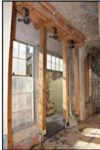
Figure 5: Powerhouse interior forming and shoring for beam repair
