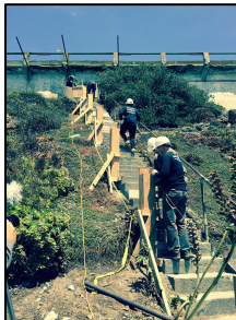
Figure 7: Recreation Yard stair repair project
