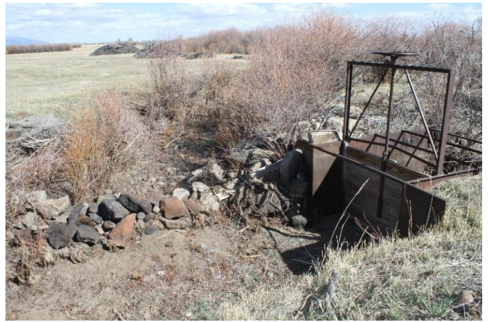
Headgate and diversion dam
