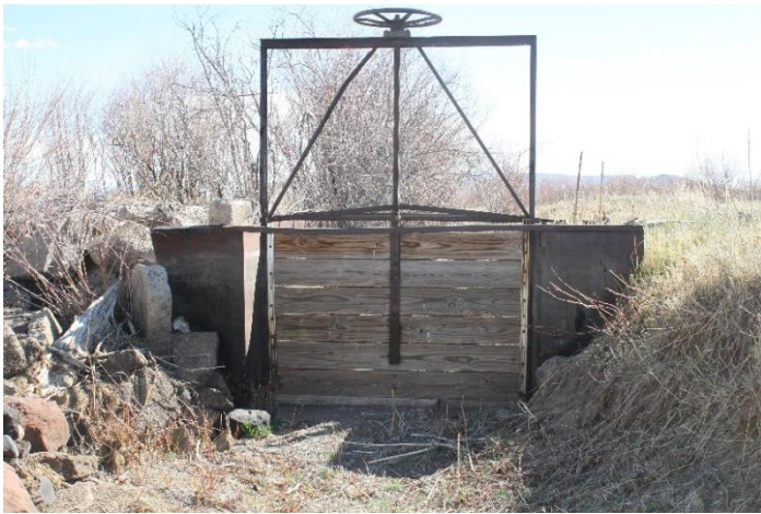
Headgate looking downstream
