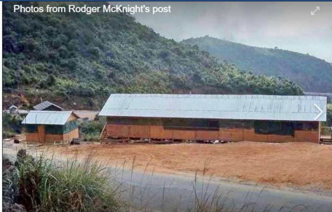
Det 2, Da Nang under construction.
