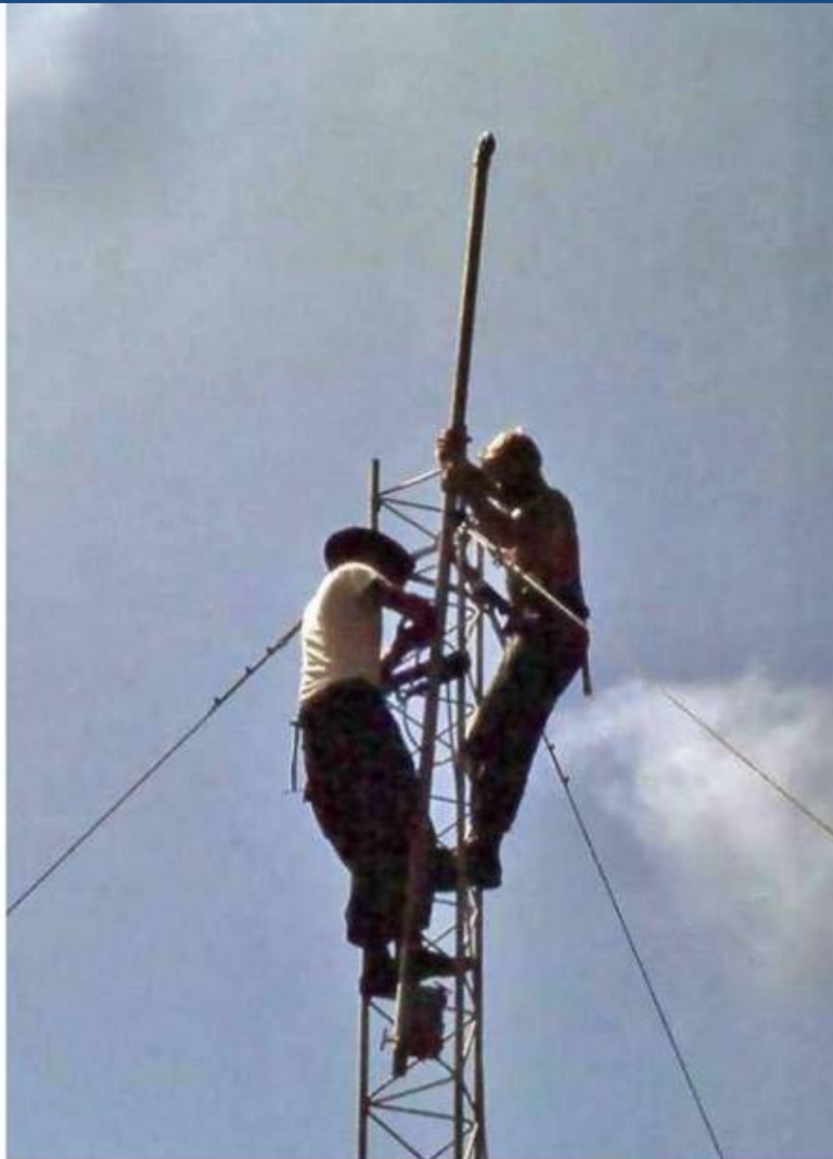
Working on the AM tower at Red Beach.
