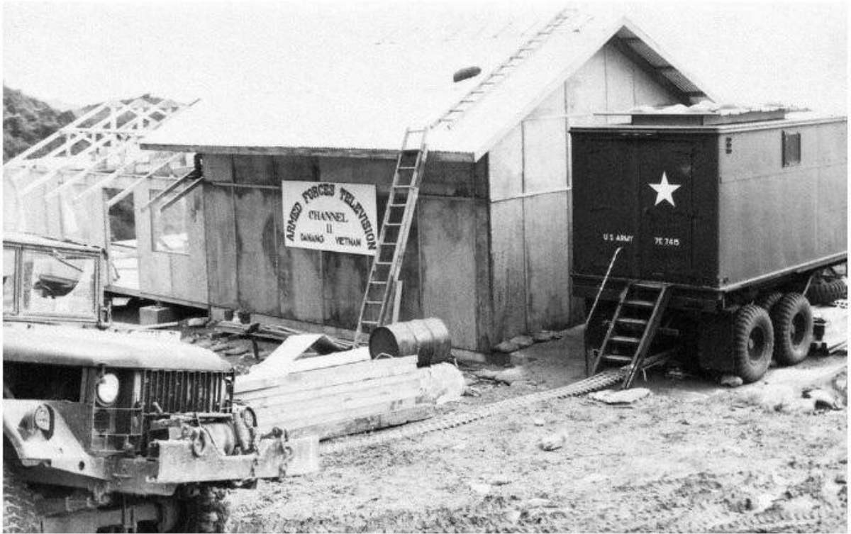
Construction of Detachment 2, Da Nang.
