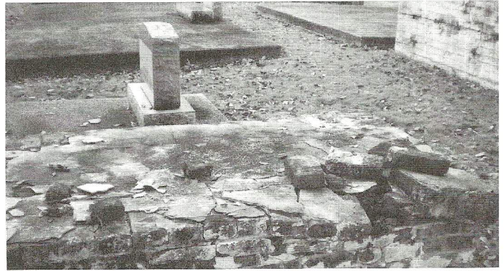
Crumbling and cracked 19th century old brick tomb
