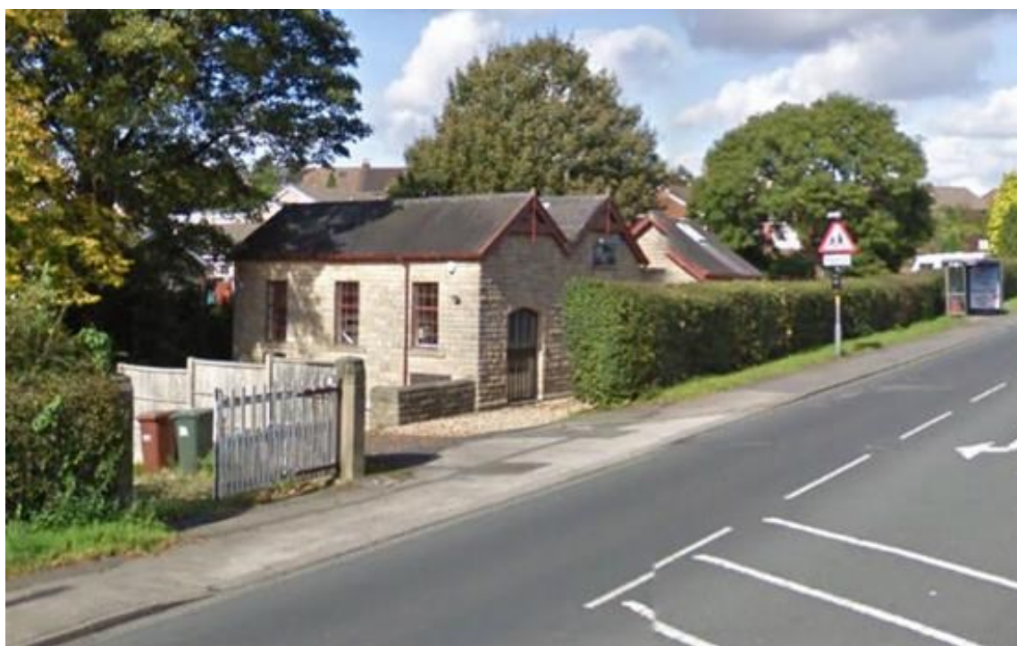
The Pumping Station on Preston Road
