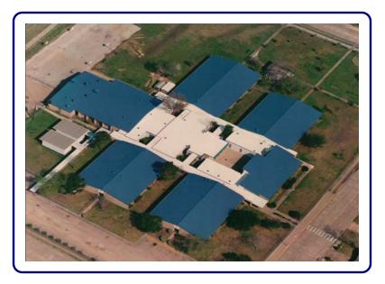
The subject facility is a functioning elementary school that was originally constructed in 1970 based on the "open-campus" concept with independent building enclosures tied together with open air covered walkways. The existing roof was a gravel-surfaced built-up roof membrane over a lightweight insulating concrete fill and metal form deck supported by open-web steel bar joists. The slopes of the roofs ranged from 1/4-inch to 1/2-inch per foot to 2-inches per foot.
