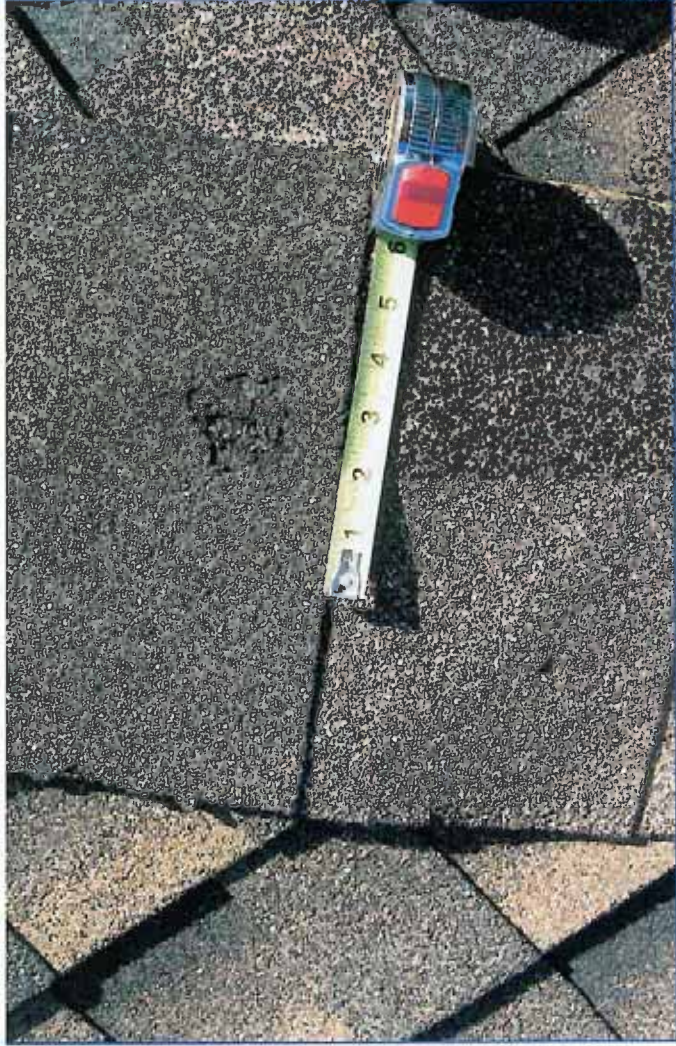
Photo 12 – Large impact on ridge shingle.
