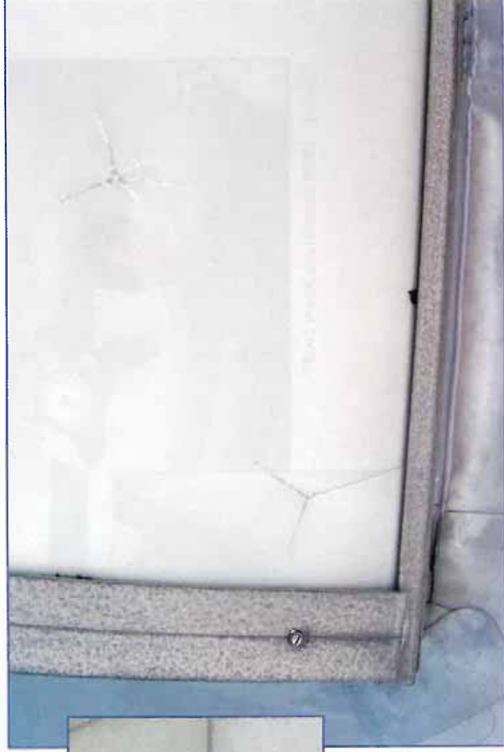
Photo 14 – Fracture in fiberglass skylight.
