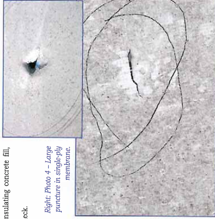
Photo 3 – Large puncture in single-ply membrane.
