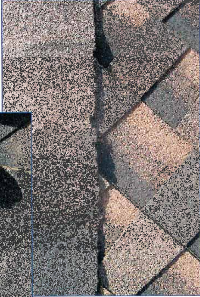
Photo 12 – Large impact on ridge shingle.
