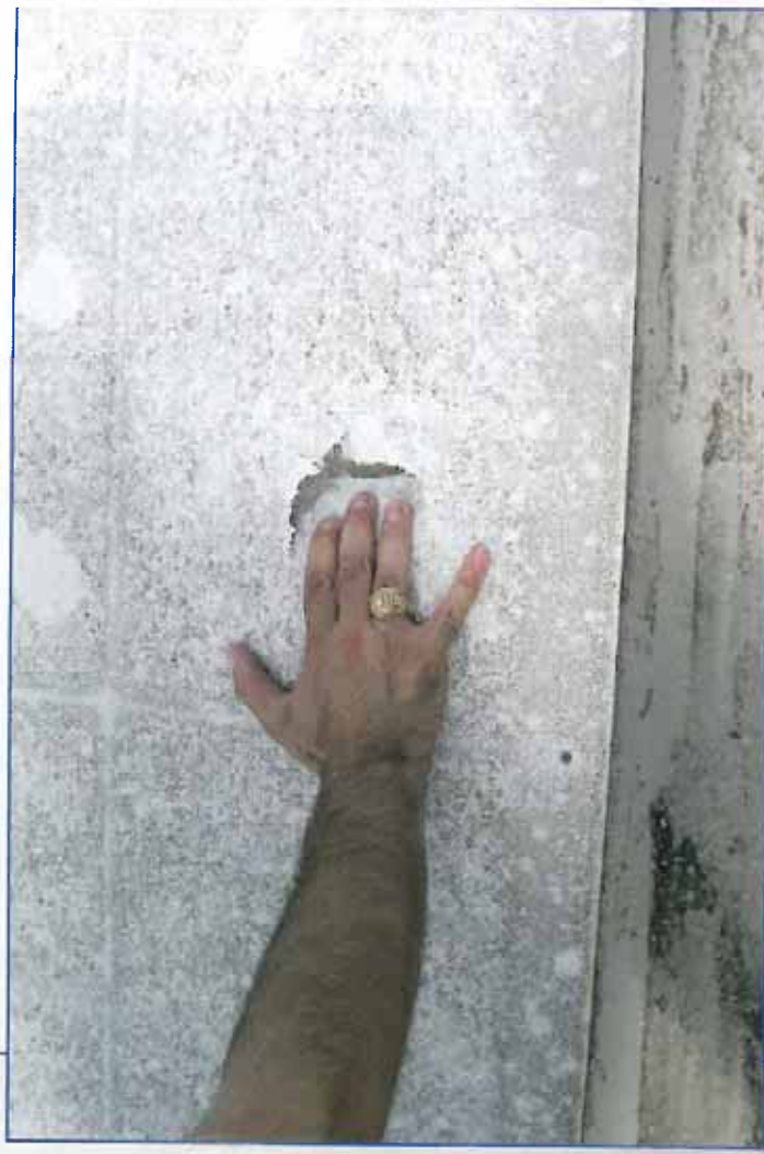
Photo 17 – Puncture in fabric skylight.
