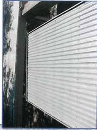
Photo 11 – Large dents in metal canopy.
