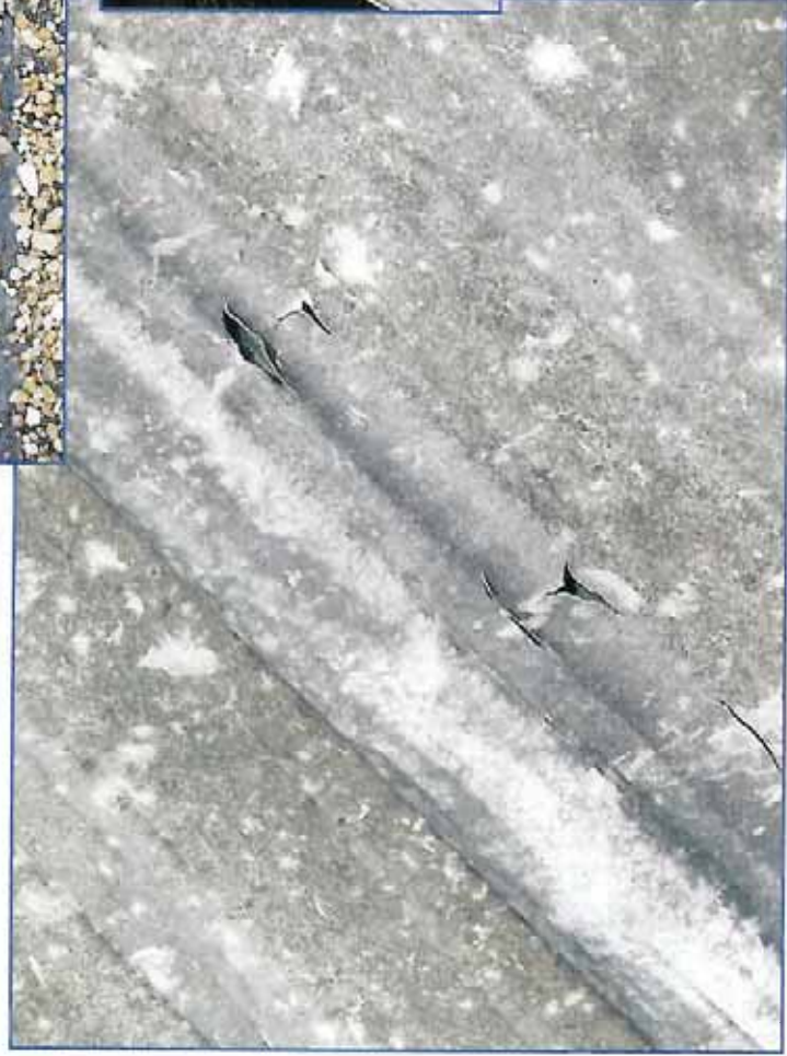
Photo 11 – Large dents in metal canopy.
