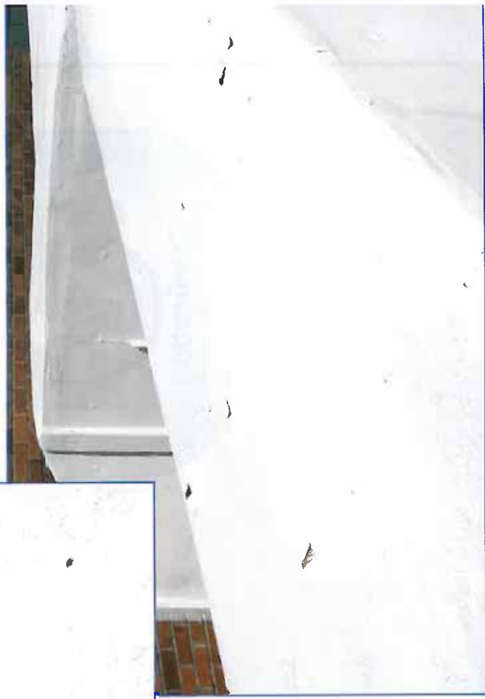
Photo 23 – Punctures in exterior insulated duct.
