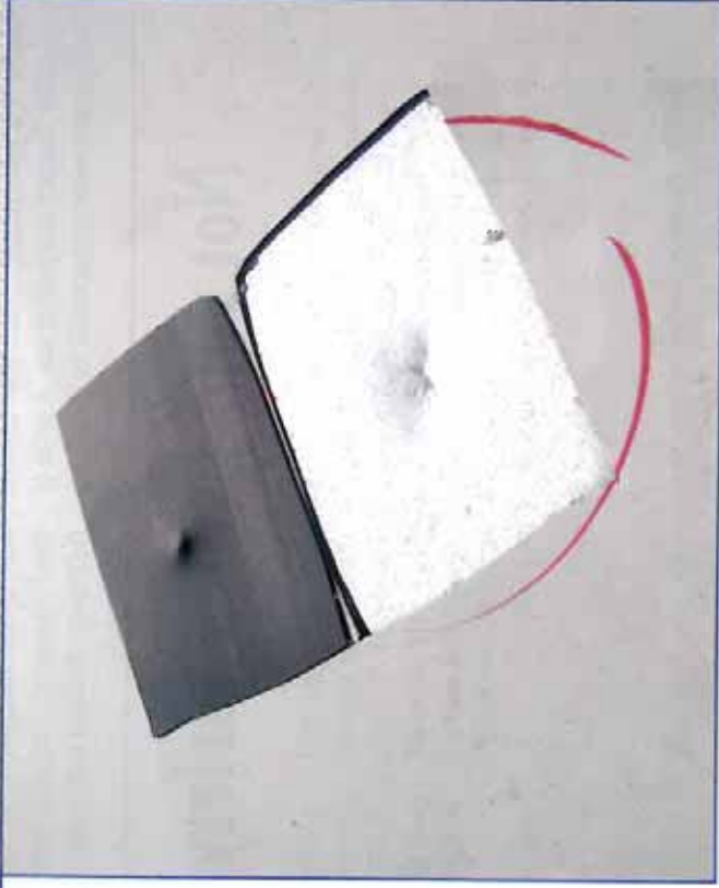
Photo 36 – Large depression in insulation board.
