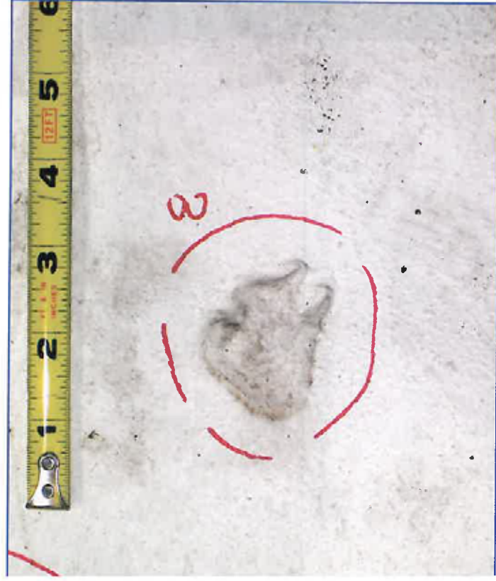
Photo 43 – Sealant and coating applied over membrane.
