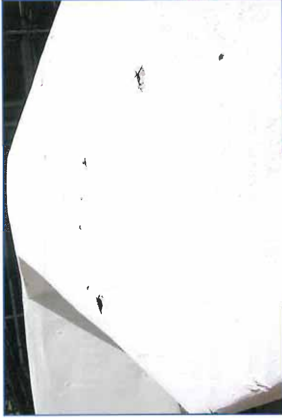
Photo 22 – Punctures in exterior insulated duct.
