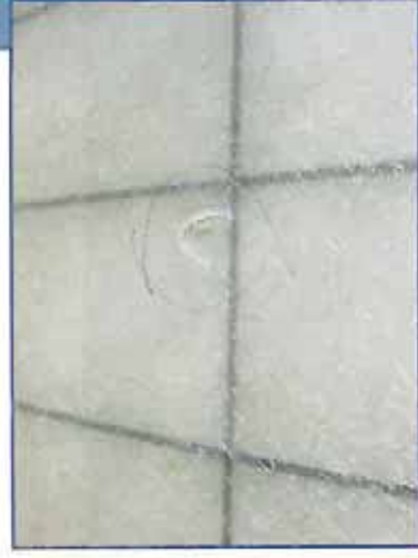
Photo 14 – Fracture in fiberglass skylight.
