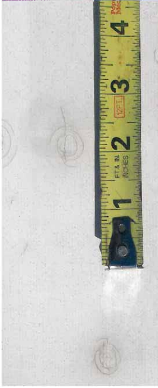
Below: Photo 6: - Spiral and linear fractures in single- ply membrane.
