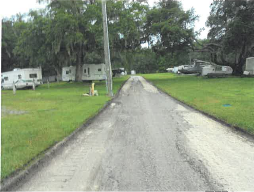
Looking at the road going into storage prior to repaving.
