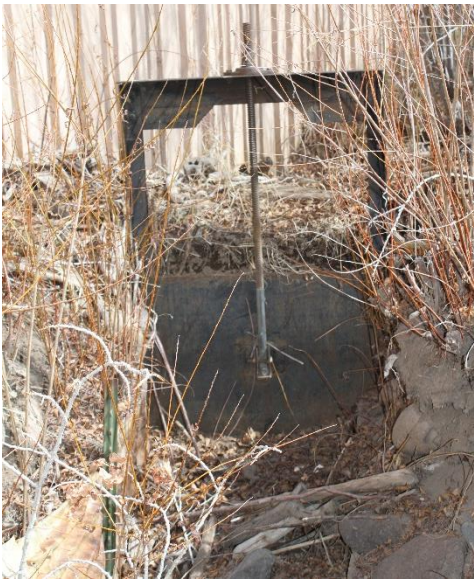
Headgate looking downstream
