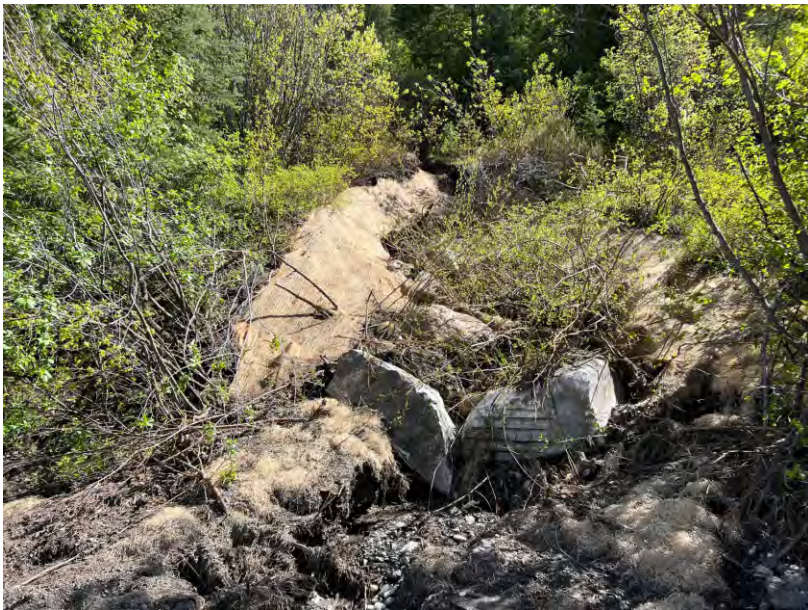
Photopoint 24. Looking south-by-southwest at erosion control measures on a seasonal drainage intersecting the main access road (6/4/23).
