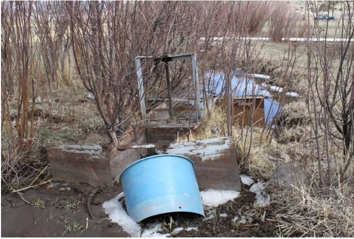
Headgate looking downstream
