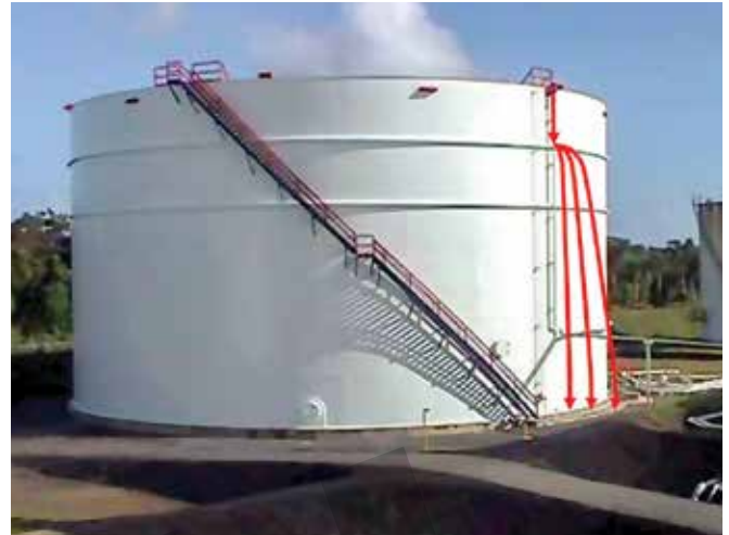
FIG. 2. Fixed-roof tank showing stiffening rings and spill trajectory into a spray cascade.
