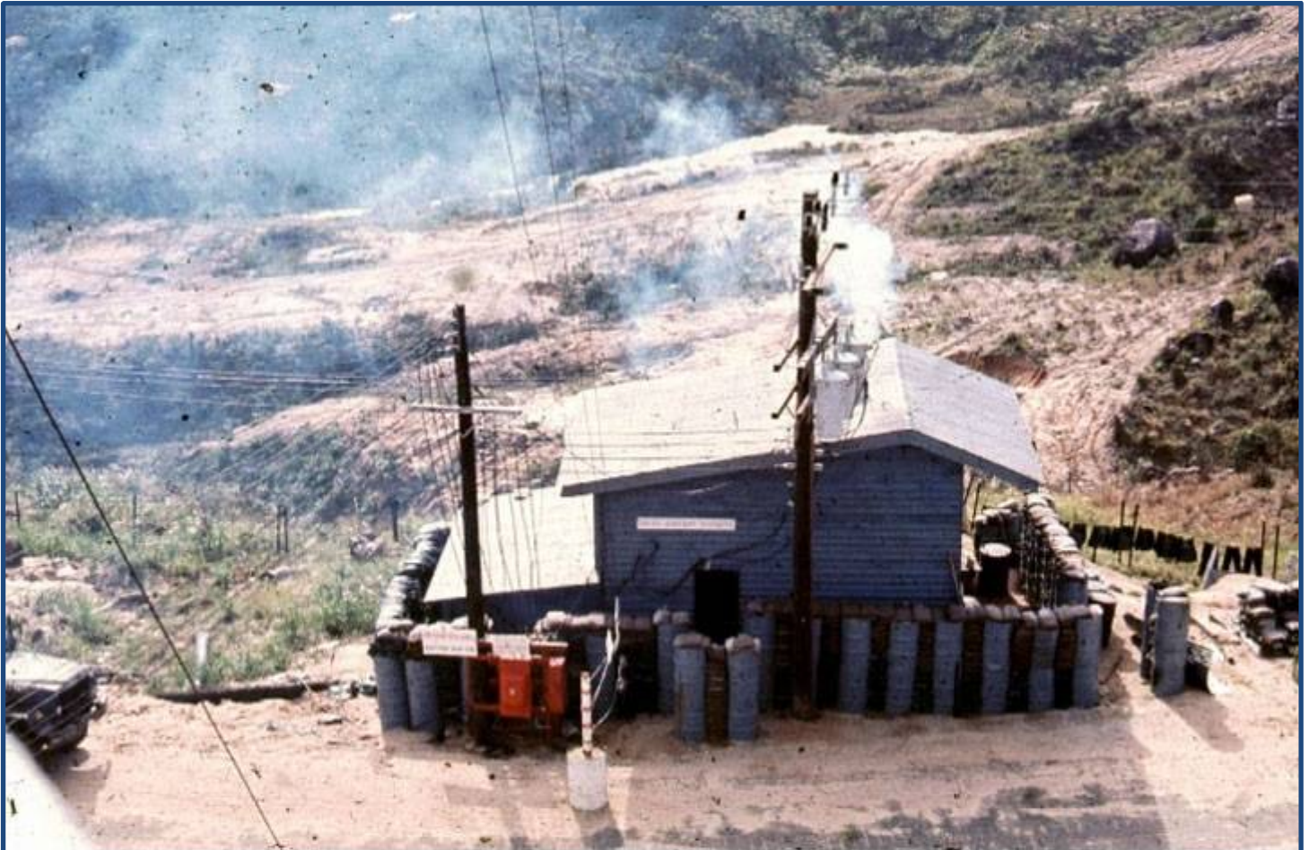
The auxiliary generator at Tuy Hoa.
