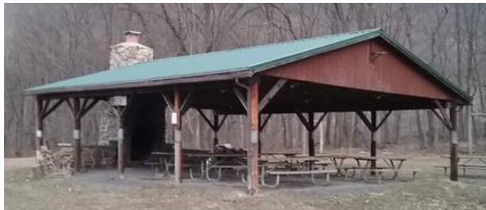
New Roof at the Pavilion
