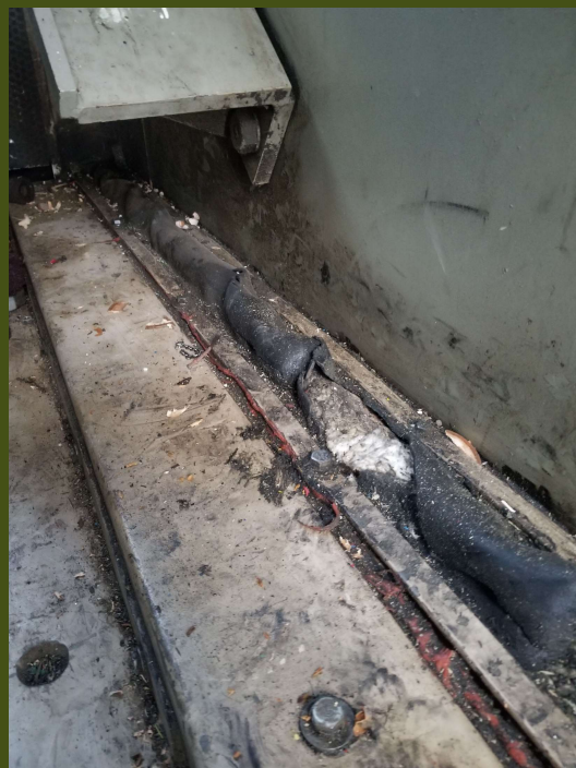
Before - Load Compartment Floor
