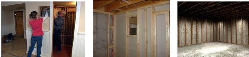
Insulating the walls with a minimum of R11 ([R value](#)) and the ceiling and floor with a minimum for R12 is what our instruction asks for. Please remember that these are min requirements you can use better insulation and get a higher R value and help the unit. Walls that have direct sun light or cold winter temperatures should have a greater insulation R value that way the wine cellar will have less change of temp in the room.
