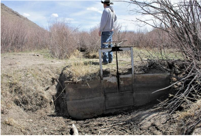
Headgate looking downstream
