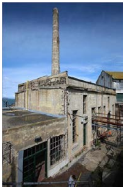
Before: Power House
