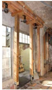
Interior façade beam formwork
