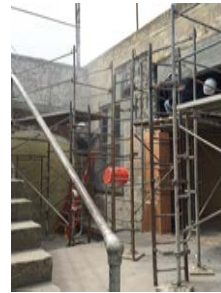
Scaffolding constructed by team at facade
