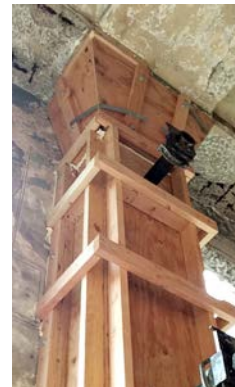
In Progress: Interior column with custom formwork for pumped concrete
