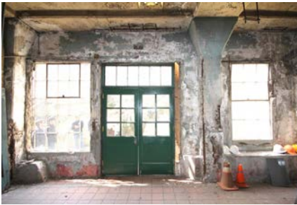
Interior façade existing conditions
