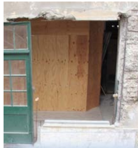
Historic window removed during construction
