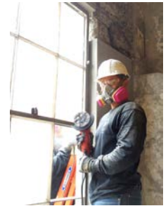
Team member grinding surface of repairs to achieve historic texture; safety first
