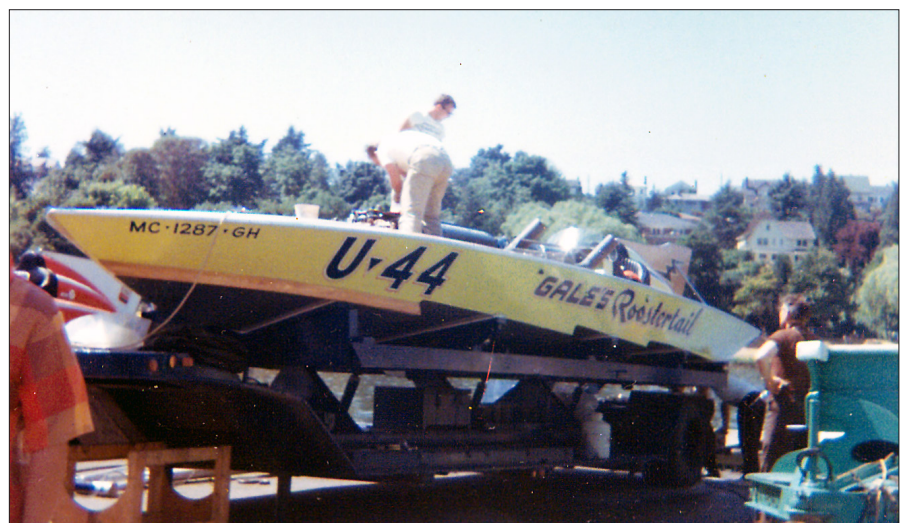
When the Gale's Roostertail was on its trailer, one could more easily see the hull's underside and the steps that pushed the boat to the water's surface.
